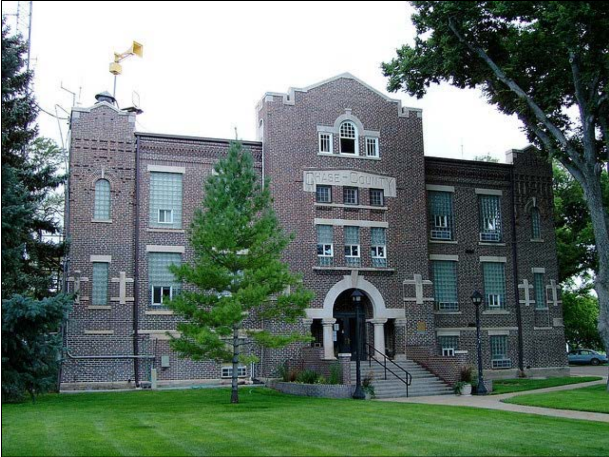
Chase County Courthouse, Imperial, NE
