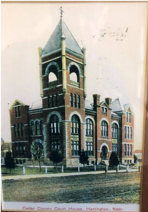
As originally built
