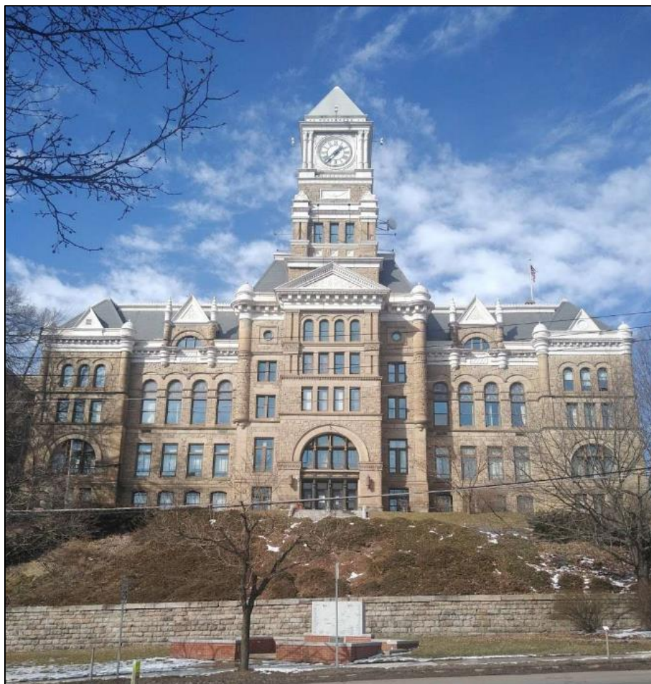
The Schuylkill County Courthouse was dedicated on September 3, 1891. It had an approximate cost of $320,000, almost $180,000 over the initial estimate.
